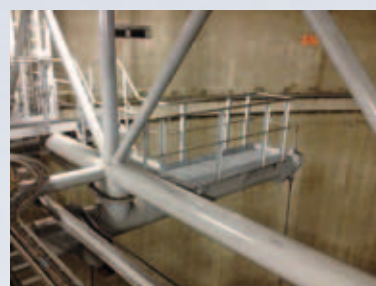
Tubular Structure to minimize dust settlement
