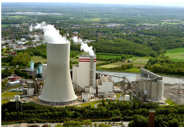
Figure 1 overview of the Lünen Coal Fired Power Plant.
