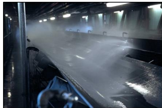
Figure 8 Spraying the Belt Conveyor under Silos
