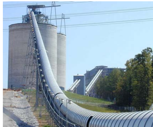
Fig. 4. Red Hills Lignite silos
