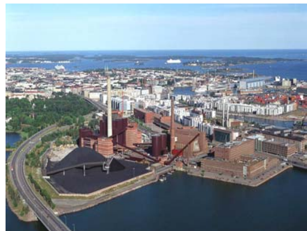
Fig. 5. Open coal storage Salmisaari Power Plant Helsinki
