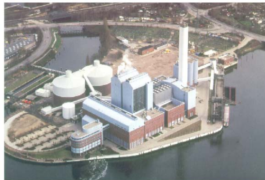
Fig. 1. The Tiefstack Power Plant in Hamburg featuring two 50,000 m 3 Eurosilos ®
