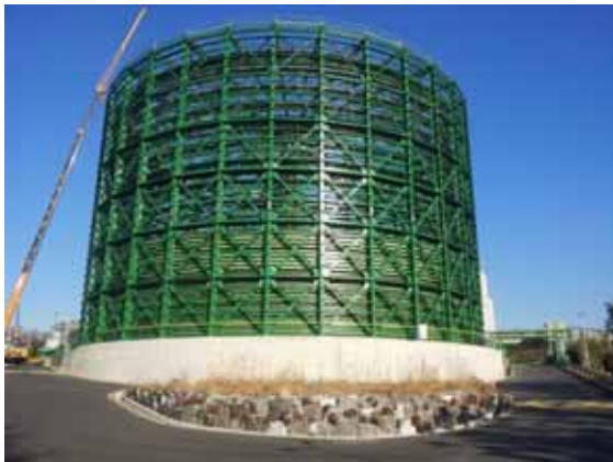
Steel structure of 40,000 Ammonium Sulfate silo
