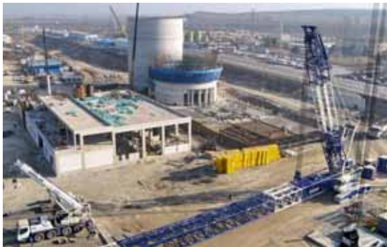
Silo slip form in progress
