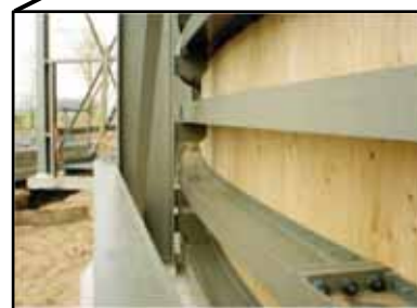
Inner wall with ring beams and wooden lining. Outer wall with standard wall cladding
