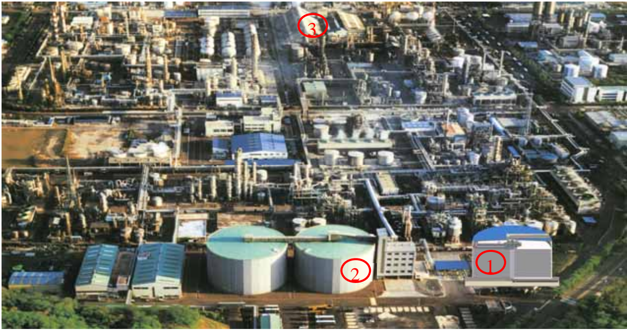
Overview silos Capro Cooperation
